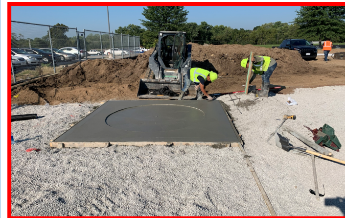
Placement of Concrete at Shotput Pads
