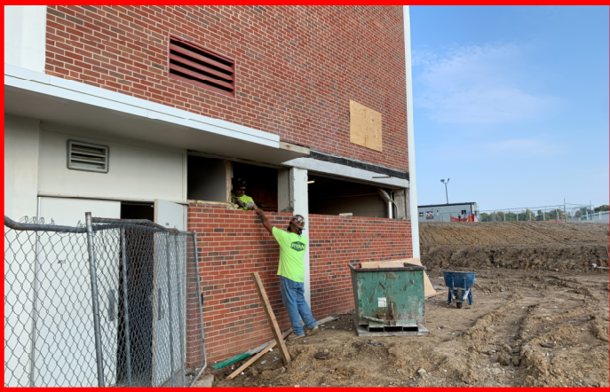
Demo/Masonry Infill at Existing Gym
