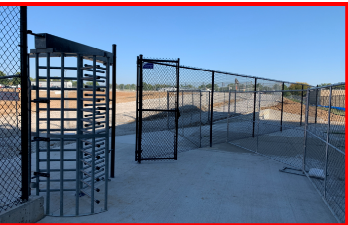
Install of Fence/Turnstile at Football Field
