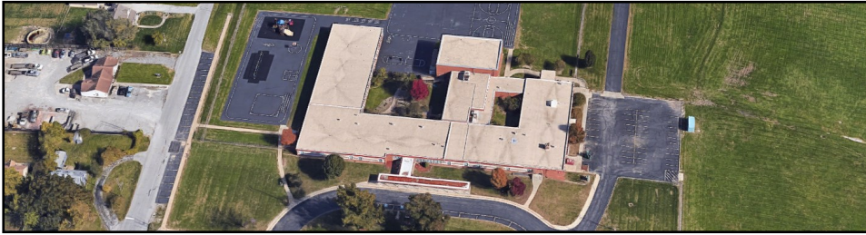
Figure 130. Aerial photo of Robinson Elementary School.
