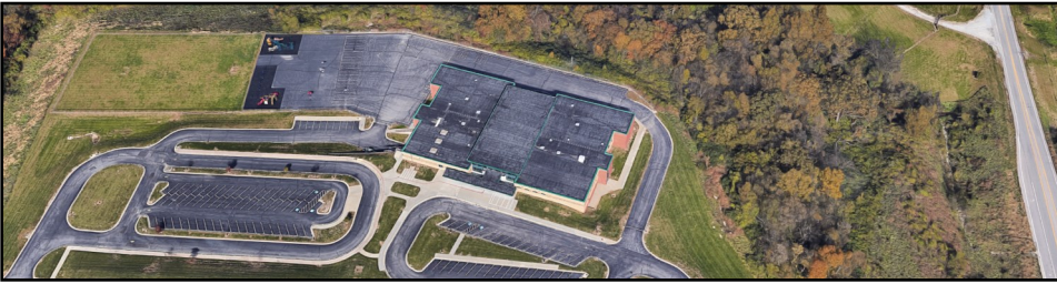
Figure 130. Aerial photo of Little Blue Elementary School.
