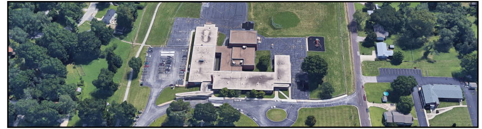
Figure 130. Aerial photo of Southwood Elementary School.
