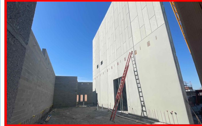
Precast Panels West Elevation of scene Shop
