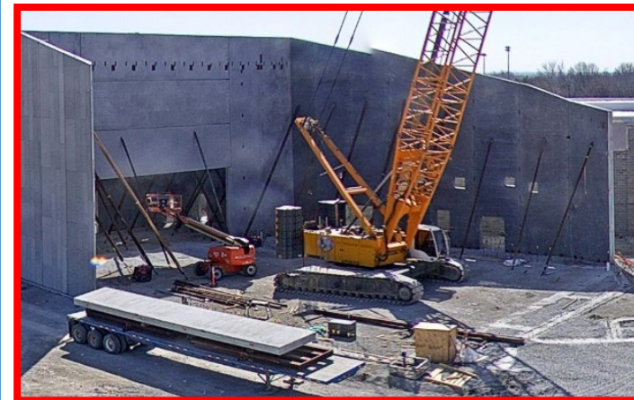
Precast Panel Status at End of Day Friday, 03/01
