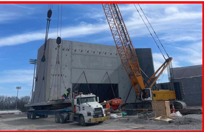
Precast Panel Erection at Stage
