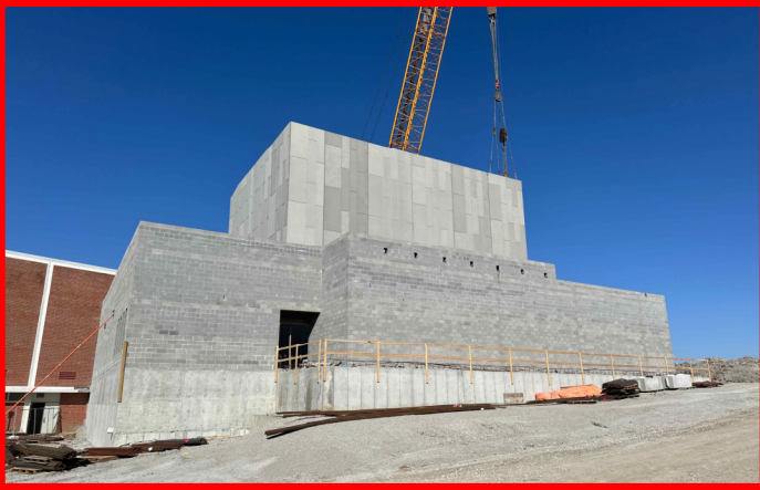
Precast Erection East Elevation of PAC
