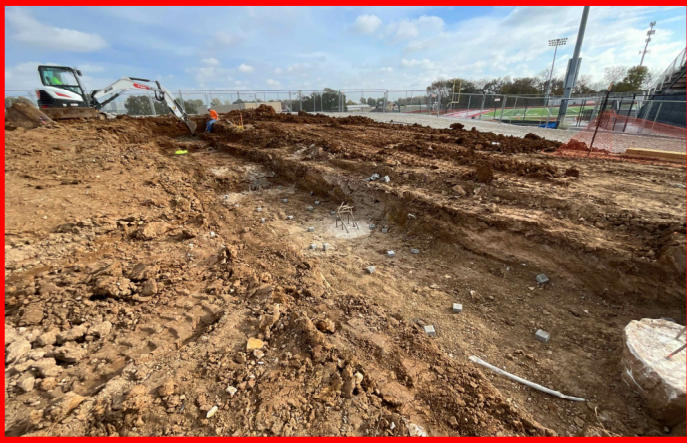
Excavate Footings East of 4' Line
