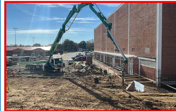
Placement of Concrete Footings
