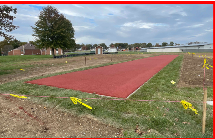
Install of Javelin Surfacing Base Layer
