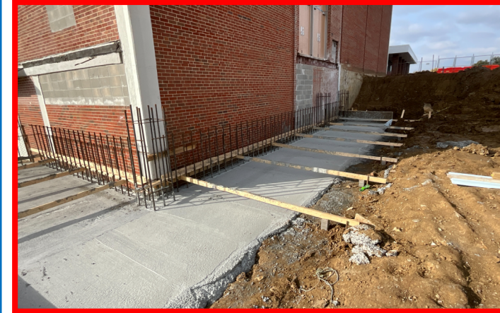
Concrete Footing Along C and A' Line
