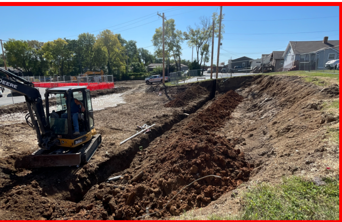
Install of Conduit for Evergy
