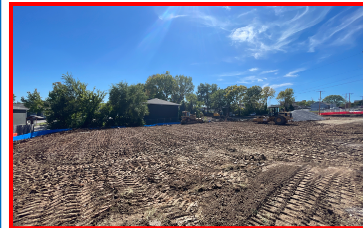
Rough Grading at East Side of site
