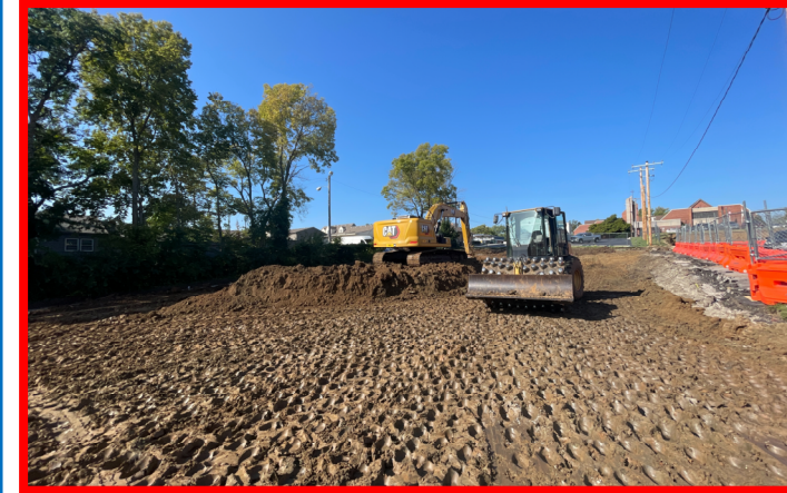
Grading at Building Pad
