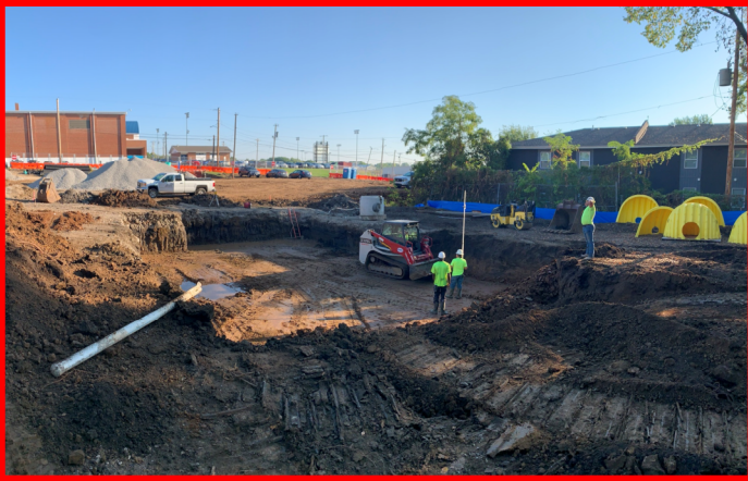
Excavation of Underground Storm System
