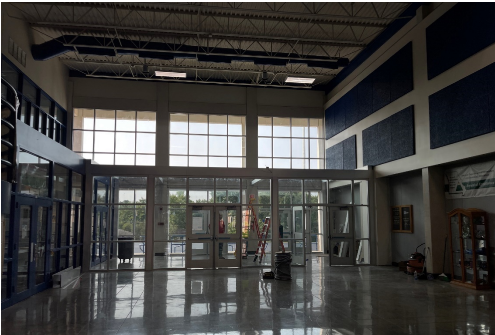
Raytown MS Secure Guided Entry Vestibule
