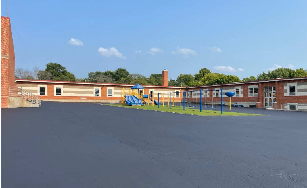
Eastwood Playground Turf and Resurfaced Asphalt
