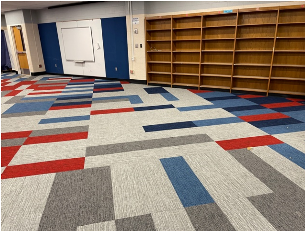
Fleetridge Media Center Finishes
