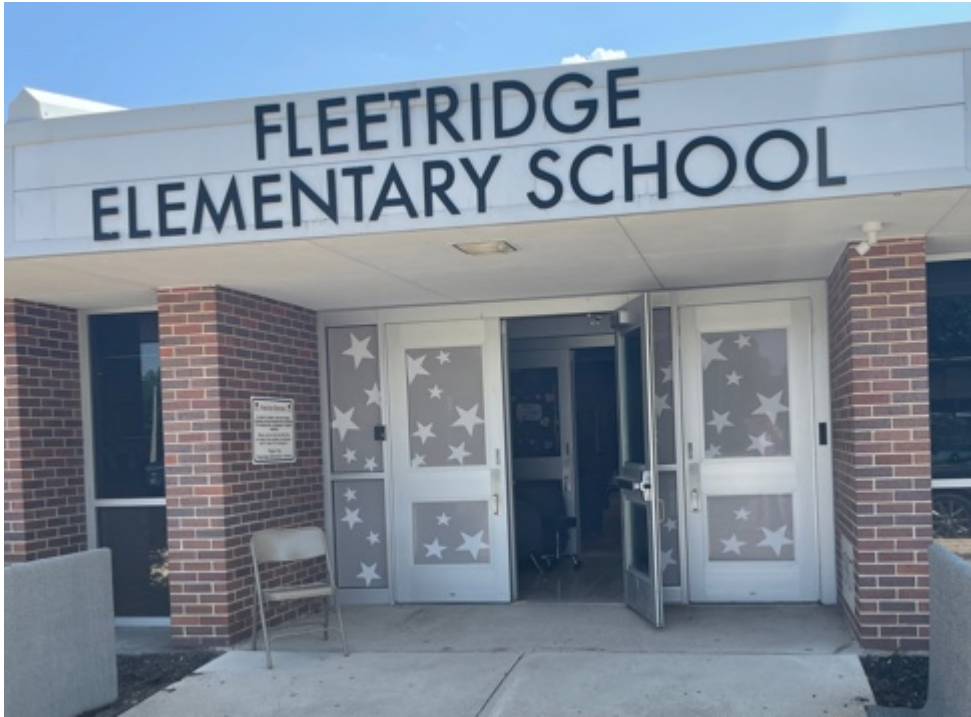
Fleetridge Elementary School Entry Glass Graphics
