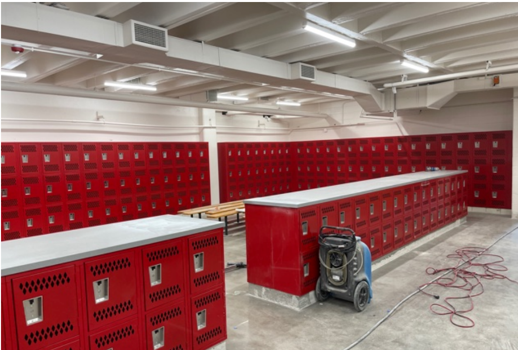
Raytown South High School Locker Room Renovations
