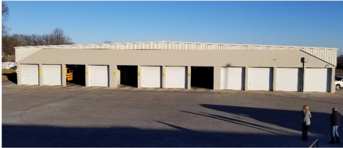
FRONT OF BUILDING
