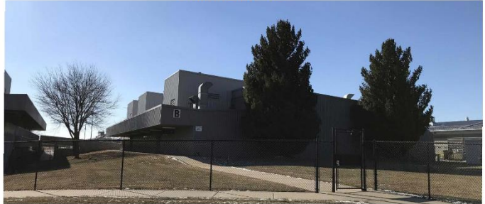
FRONT OF BUILDING
