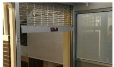
SECURE ENTRY / ACCESS CONTROL
