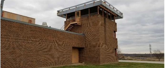
FRONT OF BUILDING
