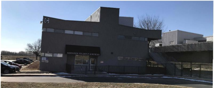
FRONT OF BUILDING
