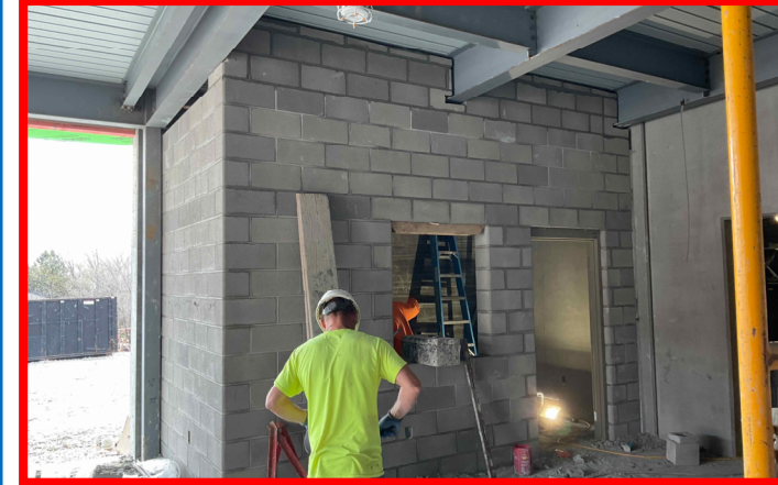
Completion of CMU Wall Install
