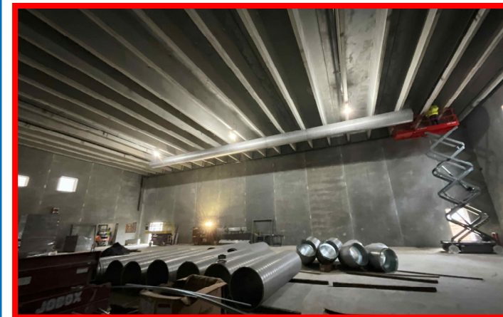
Overhead Rough In at Gym
