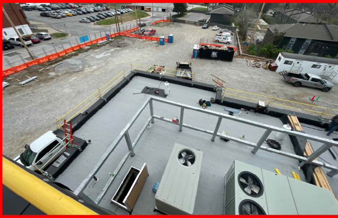
RTUs Installed and Cap Sheet Install @ Low Roof
