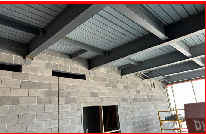
CMU Wall and Seismic Bracing Install
