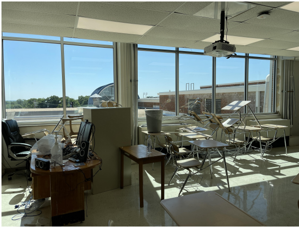
Raytown High School, New Window Installation in Progress
