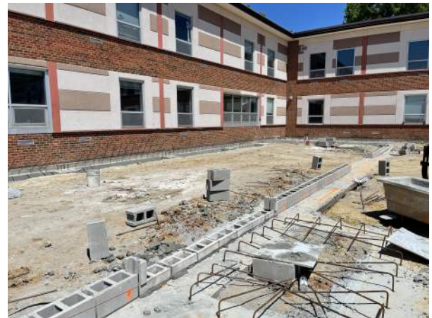
Central MS, New Addition Foundation Installed
