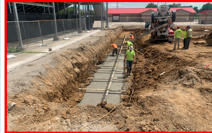
Placement of Detention Basin Footings
