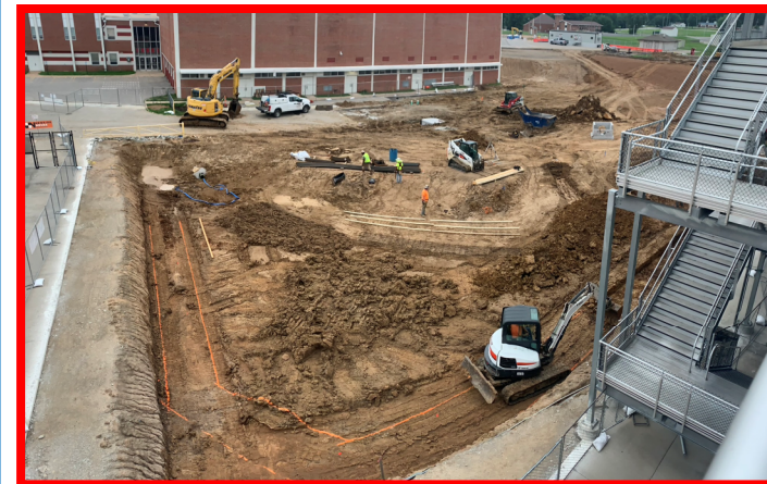
Layout/Excavation of Detention Basin Footings
