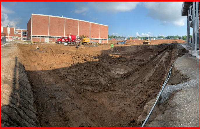
Excavation of Site Detention Basin
