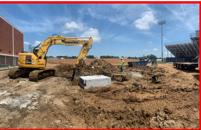
Install of Storm Drainage Structures
