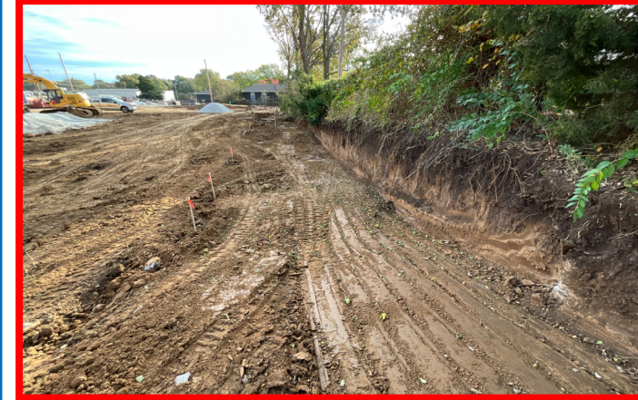
Layout and Grade for Retaining Walls
