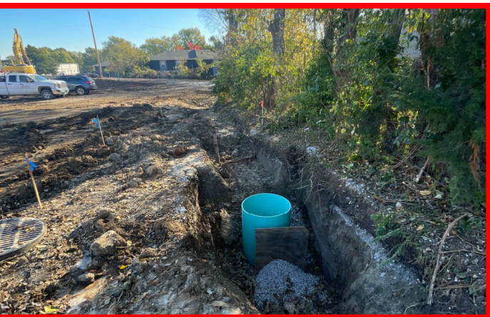
Install of Storm Structure South of Building
