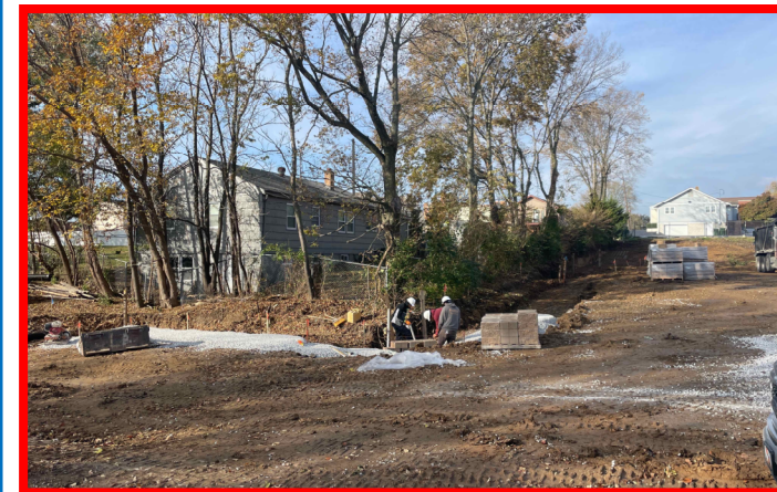
Begin Retaining Walls South of Building
