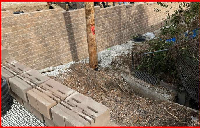
Retaining Wall SE Side of Site
