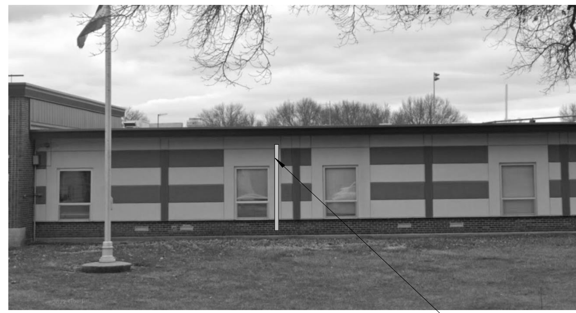
ROUTE OVERFLOW PIPE OUT EXTERIOR WALL AND TURN DOWN TO DRAIN AT 2'-0" ABOVE GRADE. VERIFY LOCATION OF EXISTING WINDOWS AND ROUTE PIPE TO MISS
