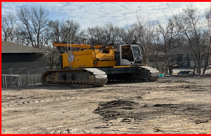
Precast Crane Mobilized
