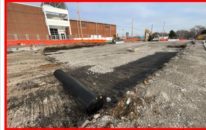
Subgrade Fix North of Building Pad
