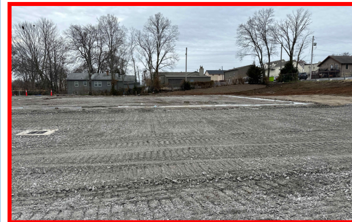
Stone Backfill at Parking/Laydown Area
