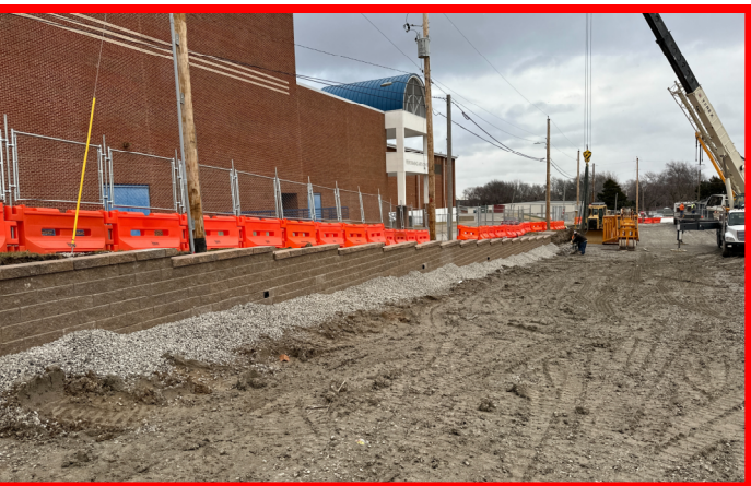
Install Complete of Retaining Wall A
