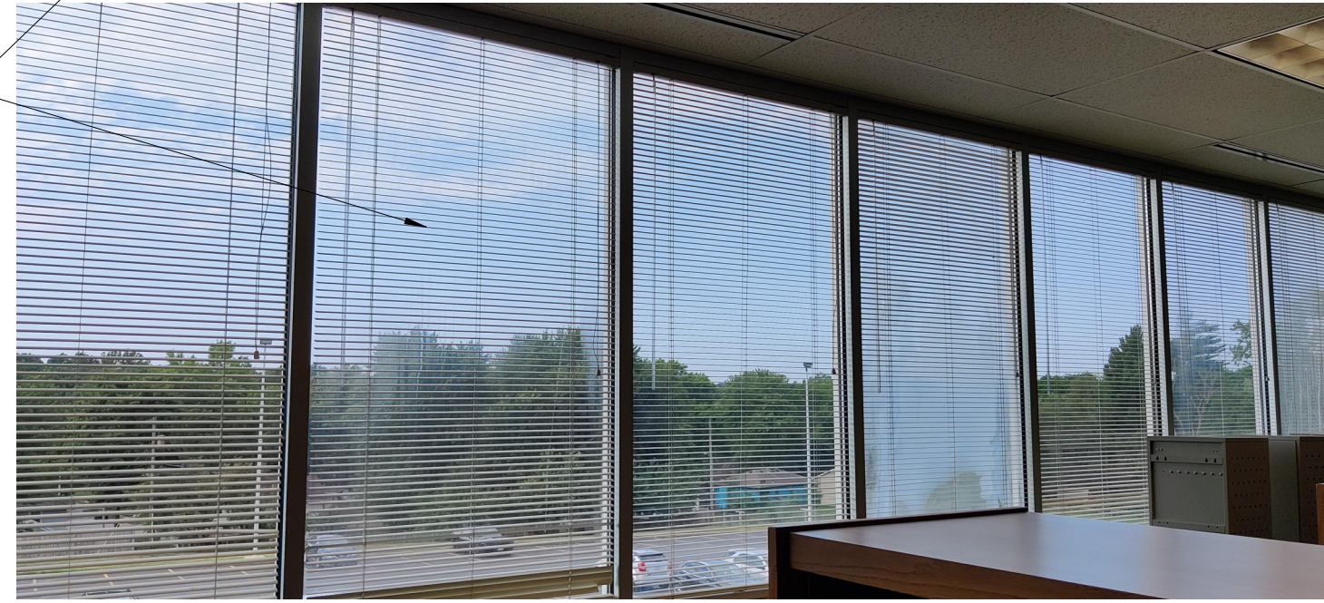
J1 Scale Media Center Glass replacement - Alternate #1
