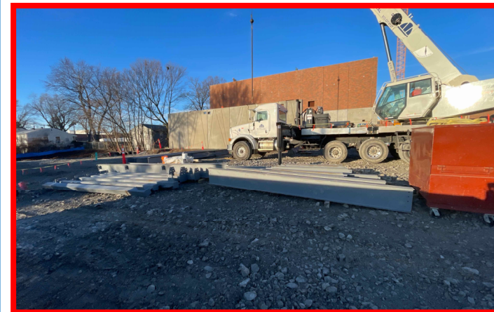
Delivery and Start of Steel
