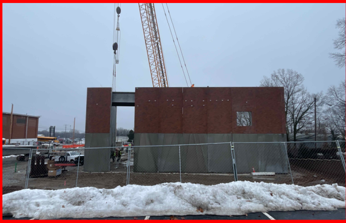
Erection of Precast West Elevation
