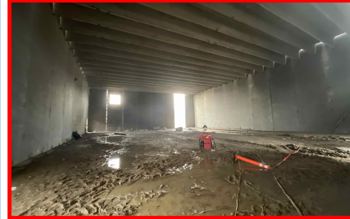
Interior View of Gym after Precast Erection
