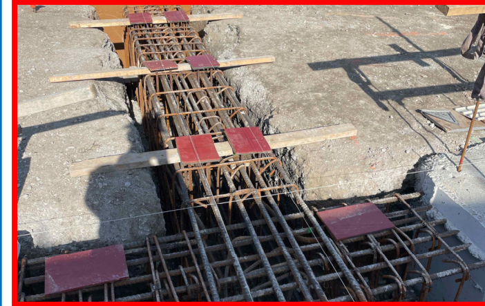
Footing Install at Back of Stage
