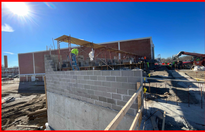
Install of CMU CL A' and 4
