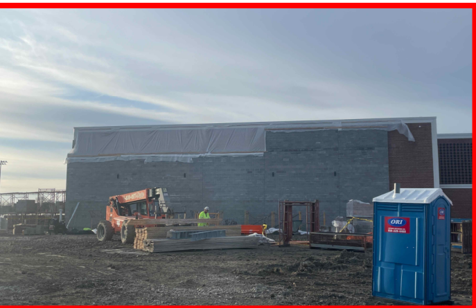
Completion of CMU Wall at CL C
