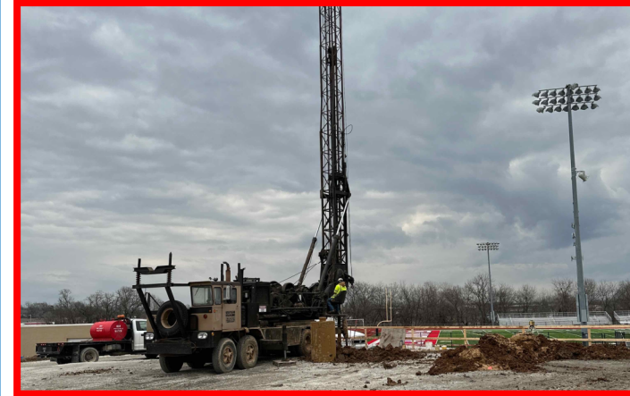
Drilling Piers at North East Corner of PAC
