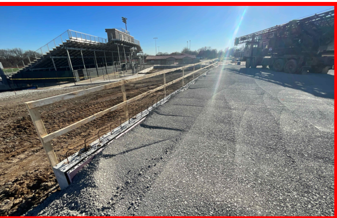
Mobilization of Pier Drill Rig
