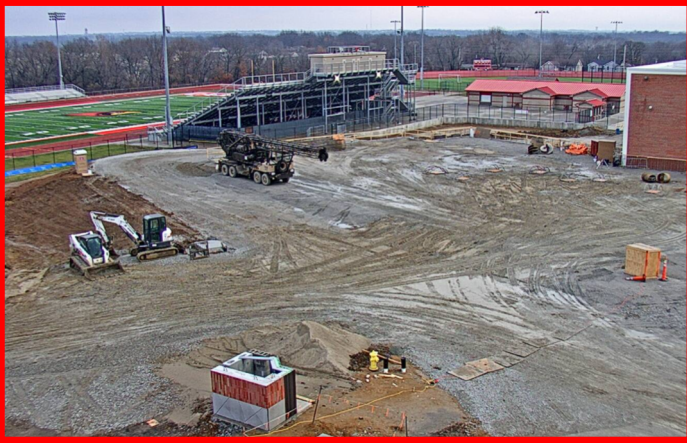
Site Conditions 12/22 Due to Weather
