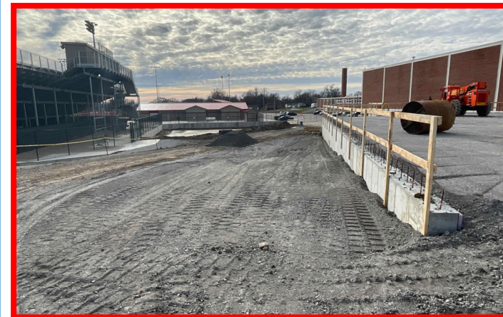
Grading/Stone Install at Perimeter of Building Pad
