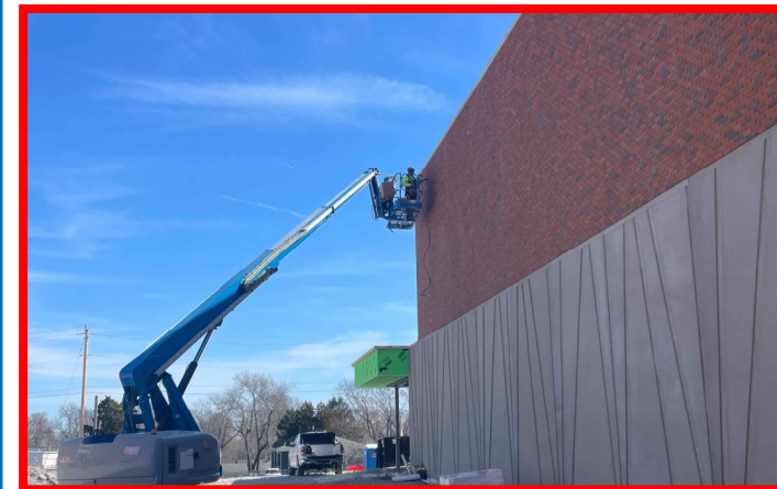
Exterior Caulking of Precast
