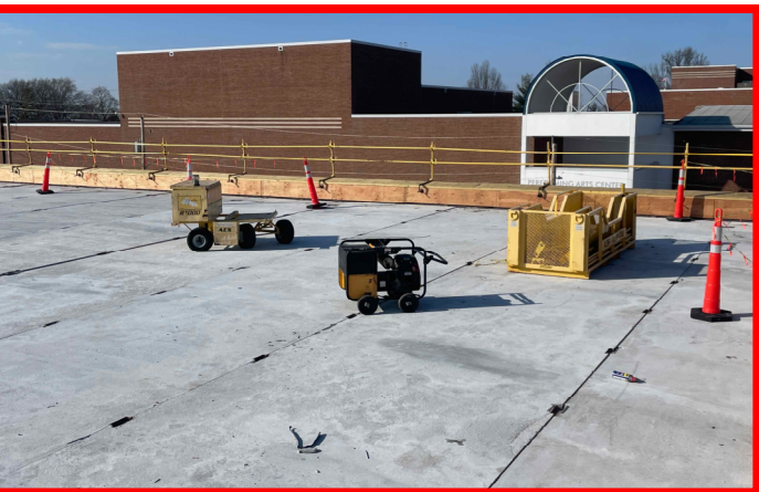
Preparation to Start Roofing
