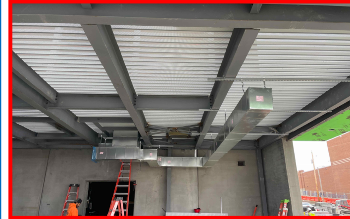
Install of Ductwork at Entrance
