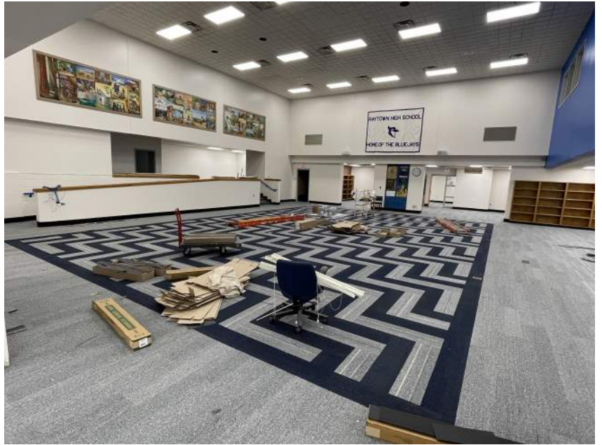
Media Center Carpet Installation, Raytown HS
